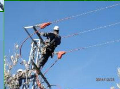
Installation without tools of the various CAON-KORWI Silicone devices. Easy to install working from the tower.
