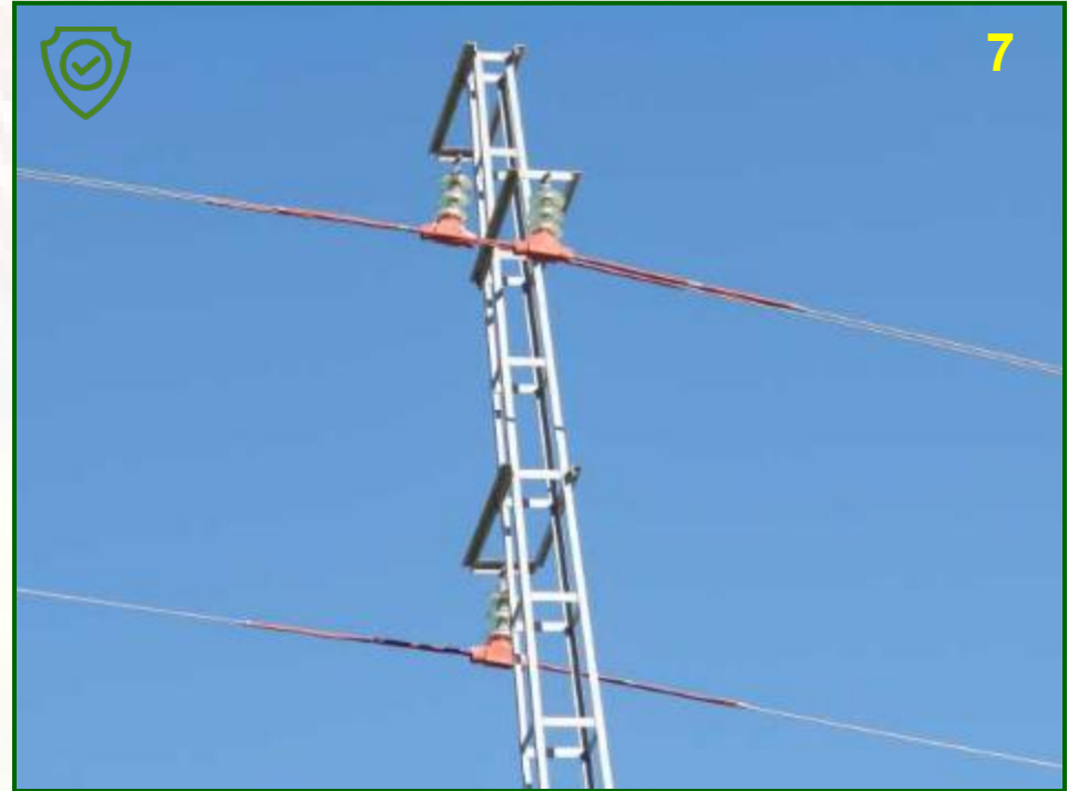
Image 5: Securing cover closure using cold vulcanising silicone tape, Mod. X-TREME by MOCAP® Image 6: Close-up view of taping on far end of clamp, without covering the SWP cover outlet to allow drainage. Image 7: Structure elements insulated in accordance with RD-1432/2008_BOJA 209.
