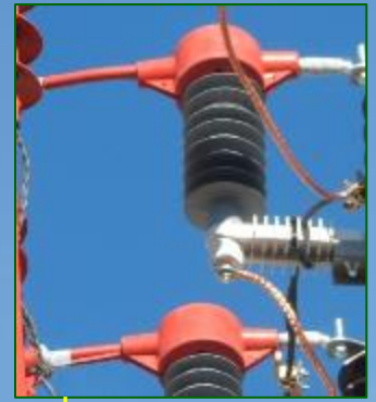
Mod. SPSA: Surge Arrester Cover with conductor entry/exit protected with Mod. SWP.
