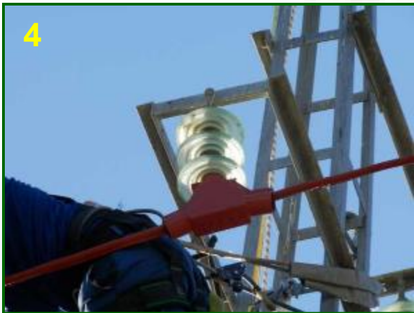
Image 2: Easy trimming, installation and closing of Mod. SWP-12 conductor cover, even at low temperatures. Image 3: Secure attachment of SWP-12 cover to the clamp by means of two (2) stainless steel ties. Image 4: Easy trimming, installation and adaptation of SPSC device to the specific application requirements. Full insulation of Ball joint and Suspension clamp.
