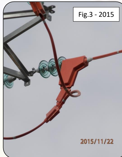
Figs. 1, 2, 3, 4 & Fig. 5: Photos taken at one-year intervals of the same deadend phase: 2013 – 2014 – 2015-2016-2017 .
