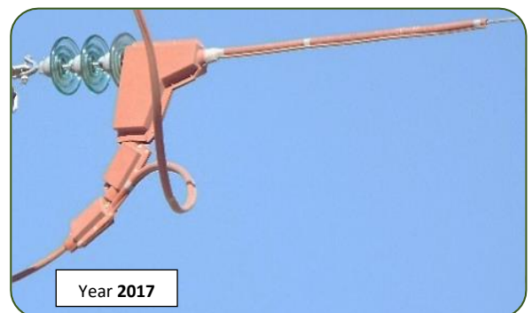
Cone-shaped sections for coupling to other cover models. Non-slipping along conductor guaranteed.
