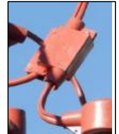
Conductor cover can adapt to small radius curves without opening up.
